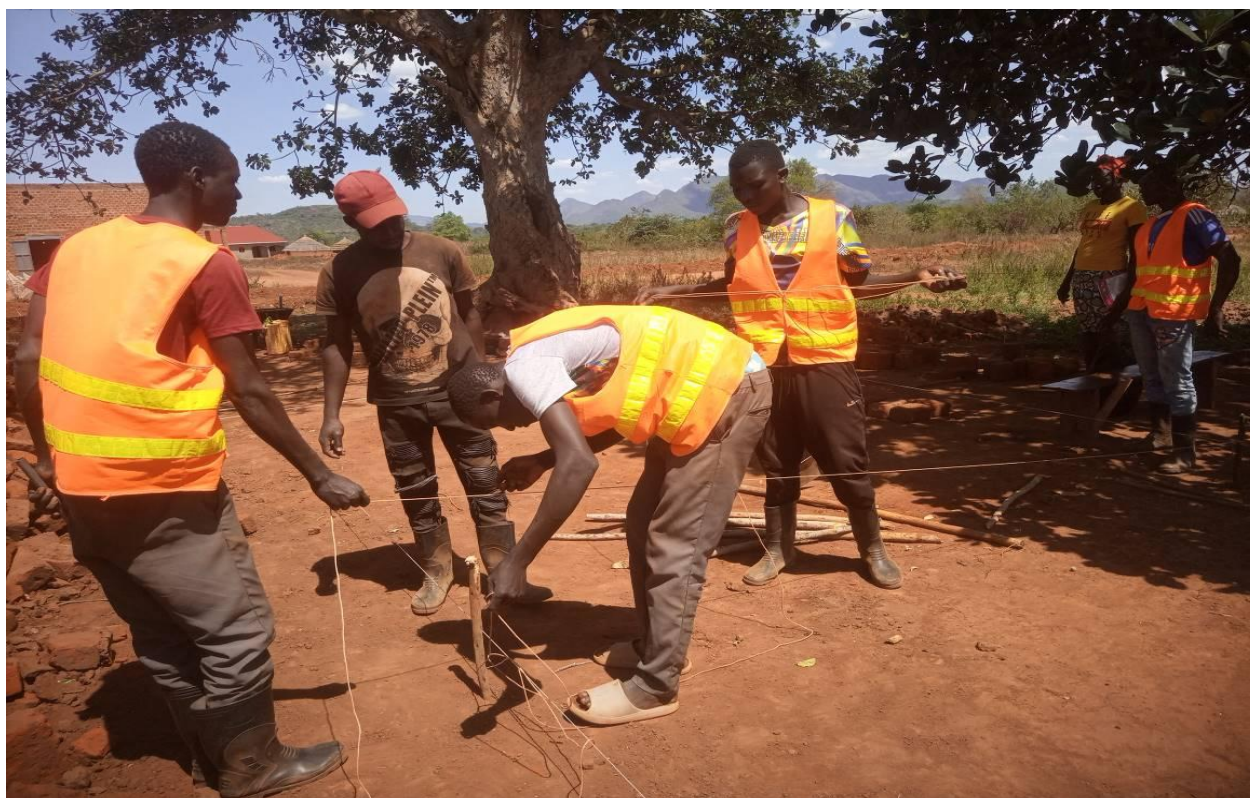
The photo above shows youth in the Community Based Training class of the skill in Brick laying and concrete practices in Adilang Agago district
